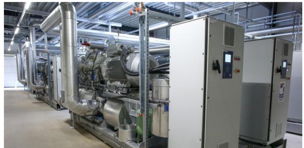
The heat pump system in Kalundborg, the unit at the front of the picture with the two electrical cabinets, forms one half of a "heat pump set". The total facility consists of a total of 6 similar units.
