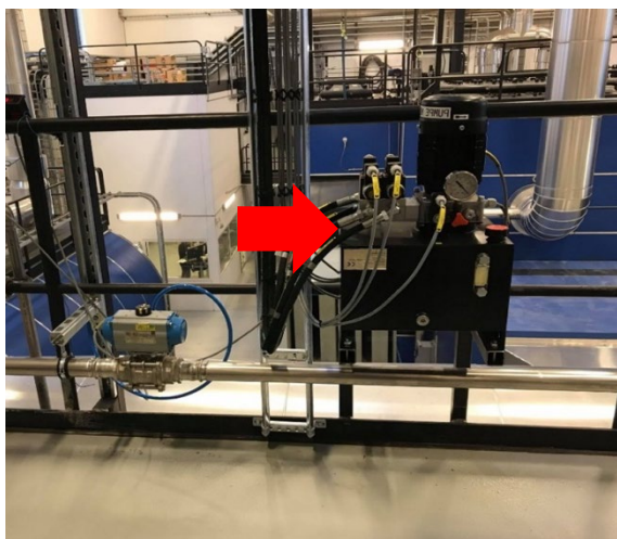
Figur 6: Hydraulisk pumpe for drift af hydraulisk cylinder.
